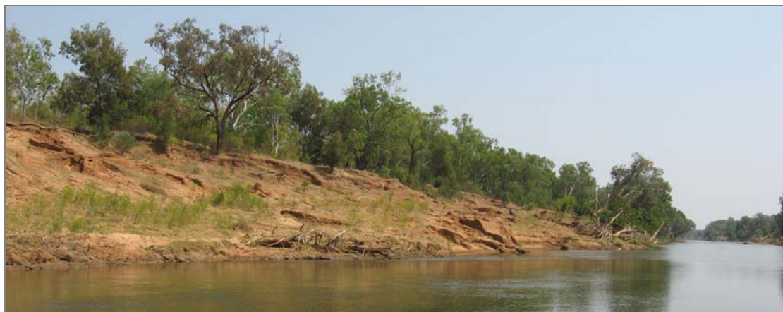
Bank erosion along the Daly river (photo courtesy of Gary Caitcheon)
